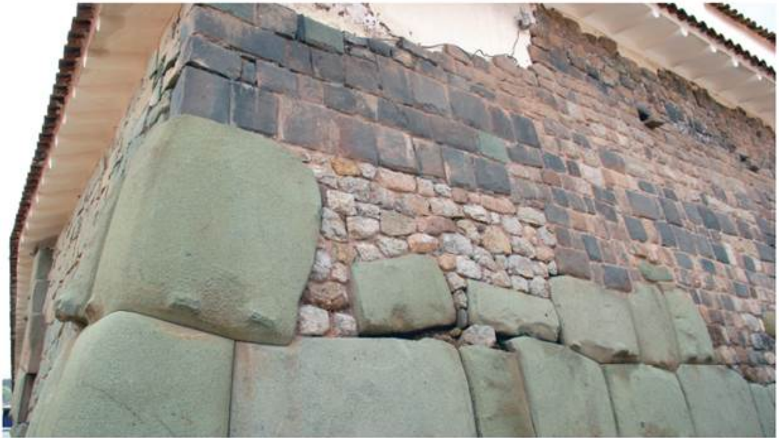
Three different building styles in the stone wall.
