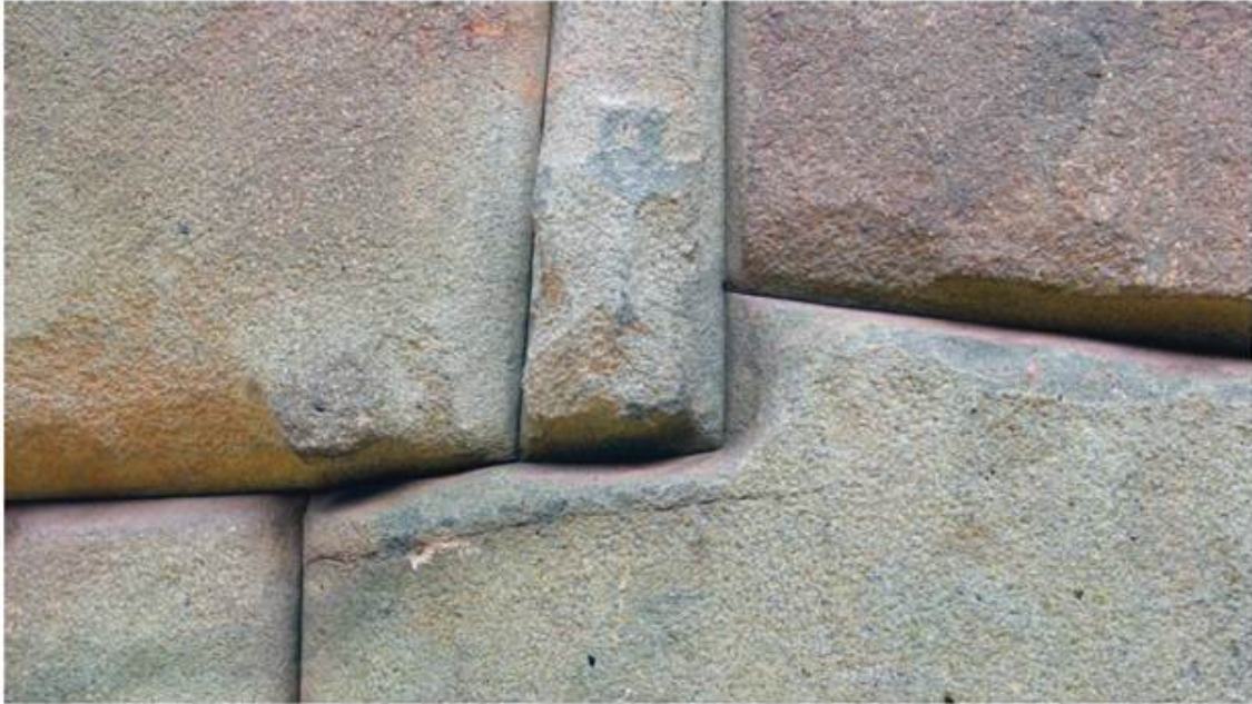
Detail from the original part of this stone wall.
