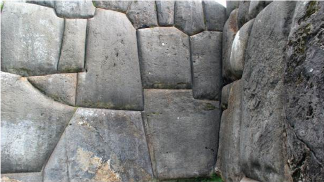
Here is a close-up so you can see the joinery.
